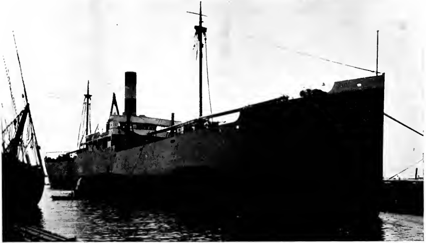
The "Thordis" laying at the wharf of her builders, the Moore and Scott Iron Works of Oakland, California. This is one of the latest of the many craft building on the Pacific Coast to be fitted with Curtis geared turbines furnished by the General Electric Company.
